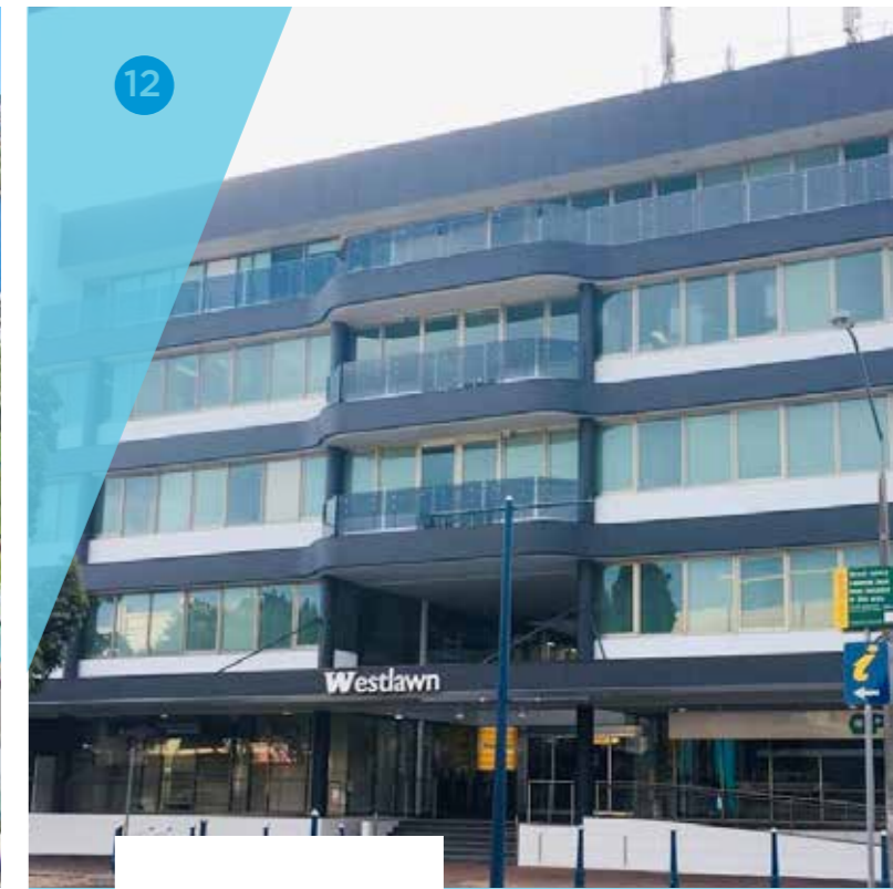
WESTLAWN BUILDING LISMORE
