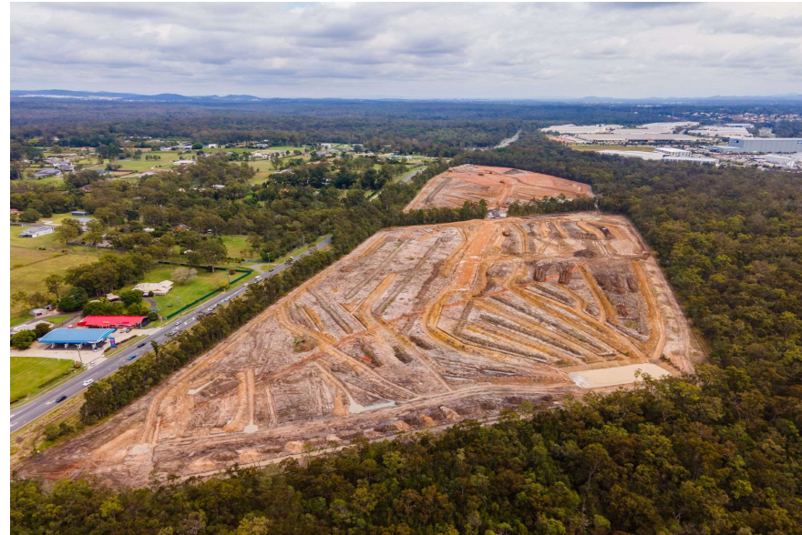
Aerial shot of 'The Hub' Heathwood, Q4 2022.
