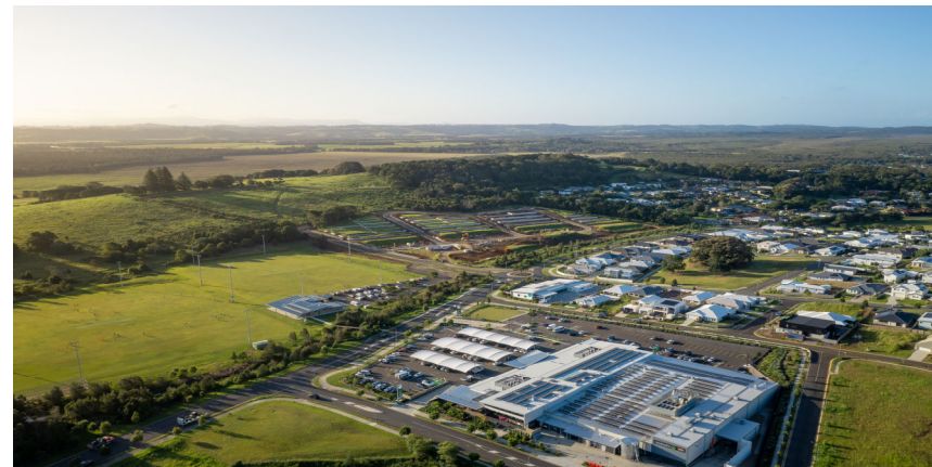
Below: Aerial shot of 'Epiq Marketplace', and 'Epiq Superlot 7' at Lennox Head.
